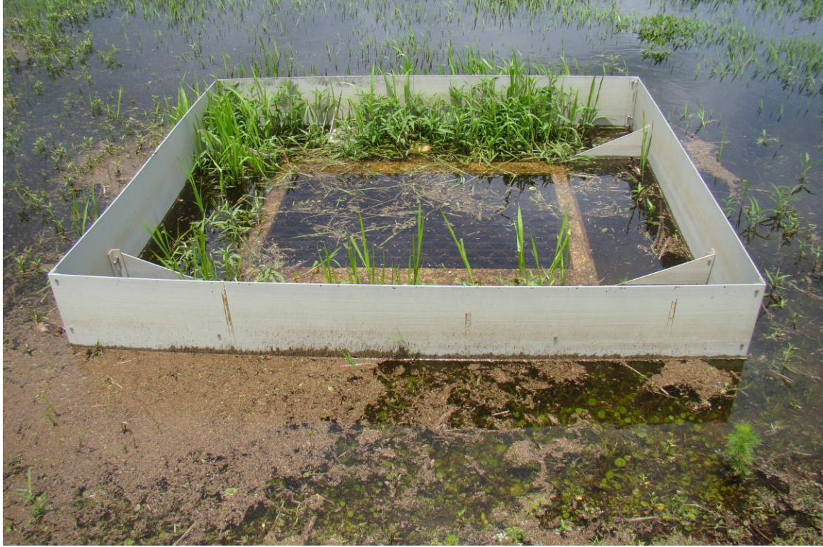
Image 3: Outfall control structure in Pond N.
