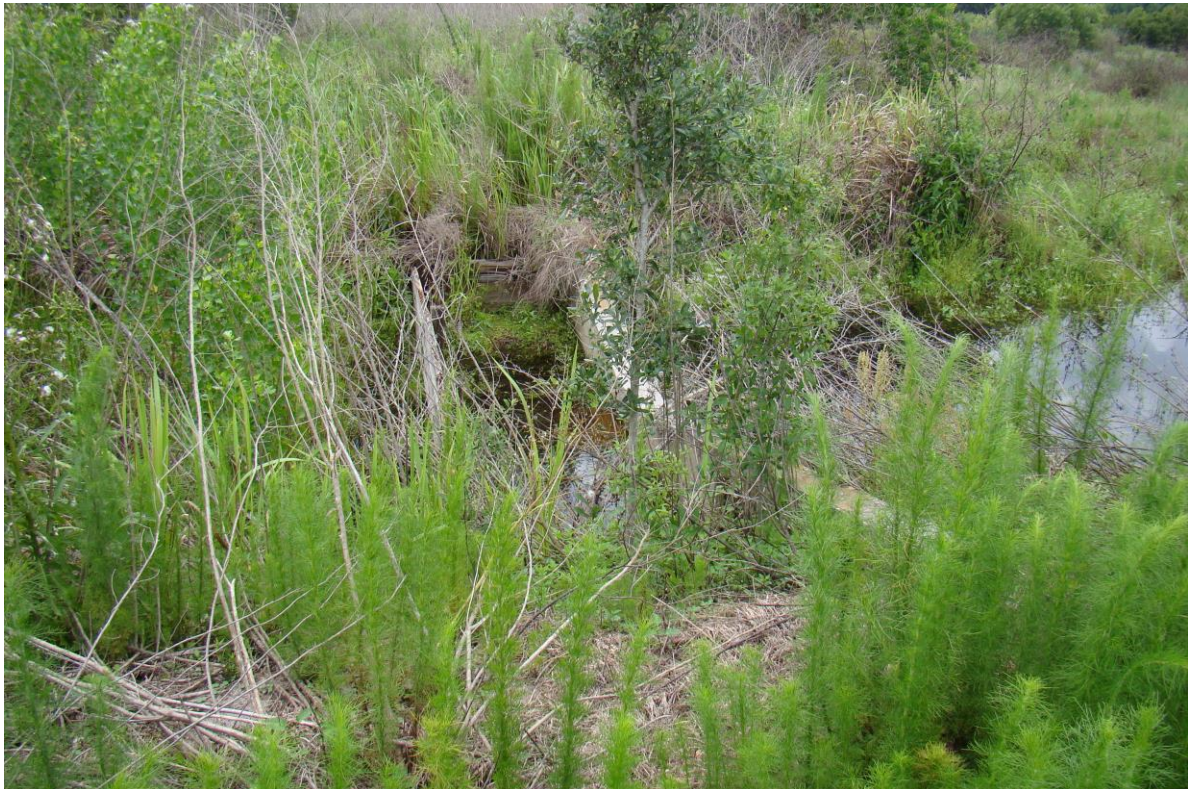
Image 6: Pond S, concrete control structure found.
