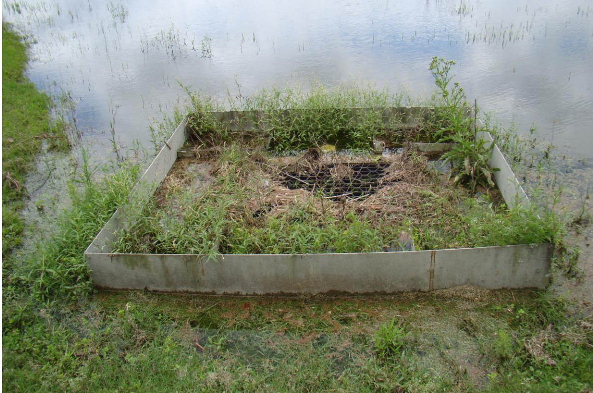
Image 1: Outfall control structure in Pond N2.
